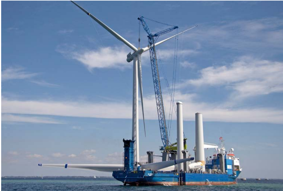
Picture 6. Installation of wind turbine at Lillgrund (Photo: Hans Blomberg/Vattenfall).
